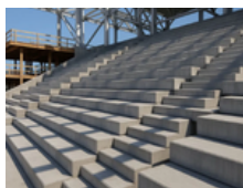
Stadium Terracing & Seating
